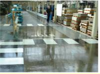
the coating into a solid film, at the same time creating a strong bond to the substrate. This fast cure eans there was minimal disruption to production as, within minutes, the floor could be used again. The floor coating is non-flammable, low odour, contains no solvents or isocyanates and complies with all the latest VOC and HAP regulations. It is designed for use on any new or
