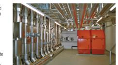
The 500kW and 1000kW models are also available in 8 bar versions. Featuring Hoval's Ultra Clean combustion system, the boilers use a modulating pre-mix down firing burner with up to 6:1 turndown (12:1 on twin units) and a stainless steel combustion chamber with a single pass aluFer tube heat exchanger. The aluFer tubes are also made of stainless steel with an aluminium alloy finned internal surface to provide a high surface area for heat exchange Tel: 01636 672711
