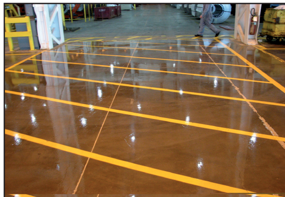
After, Safety Entrance
